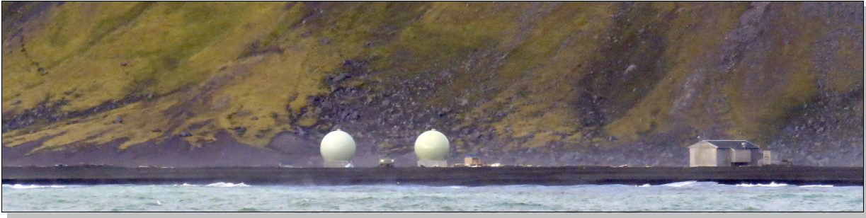
Installations Galileo, etc. (restricted area)
